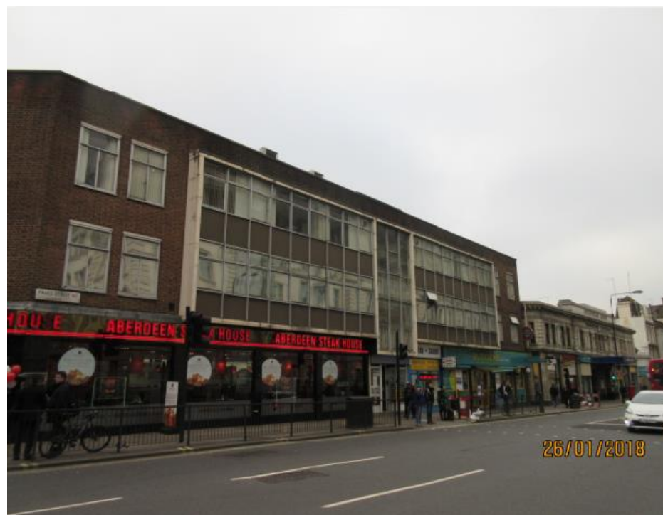
Views of existing building from Praed Street.
