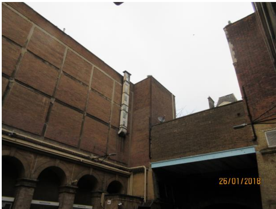
View from London Street (top) and view from existing retaining wall to Paddington District and Circle Line Underground Station as seen from platform level (bottom).
